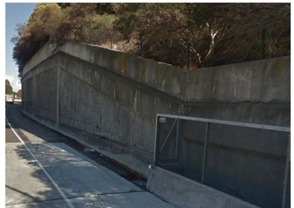
Above: Eastbound I-580 requires widening in Contra Costa County to accommodate the 3rd eastbound lane. The retaining wall shown must be removed and replaced with a wall set further back from I-580.
