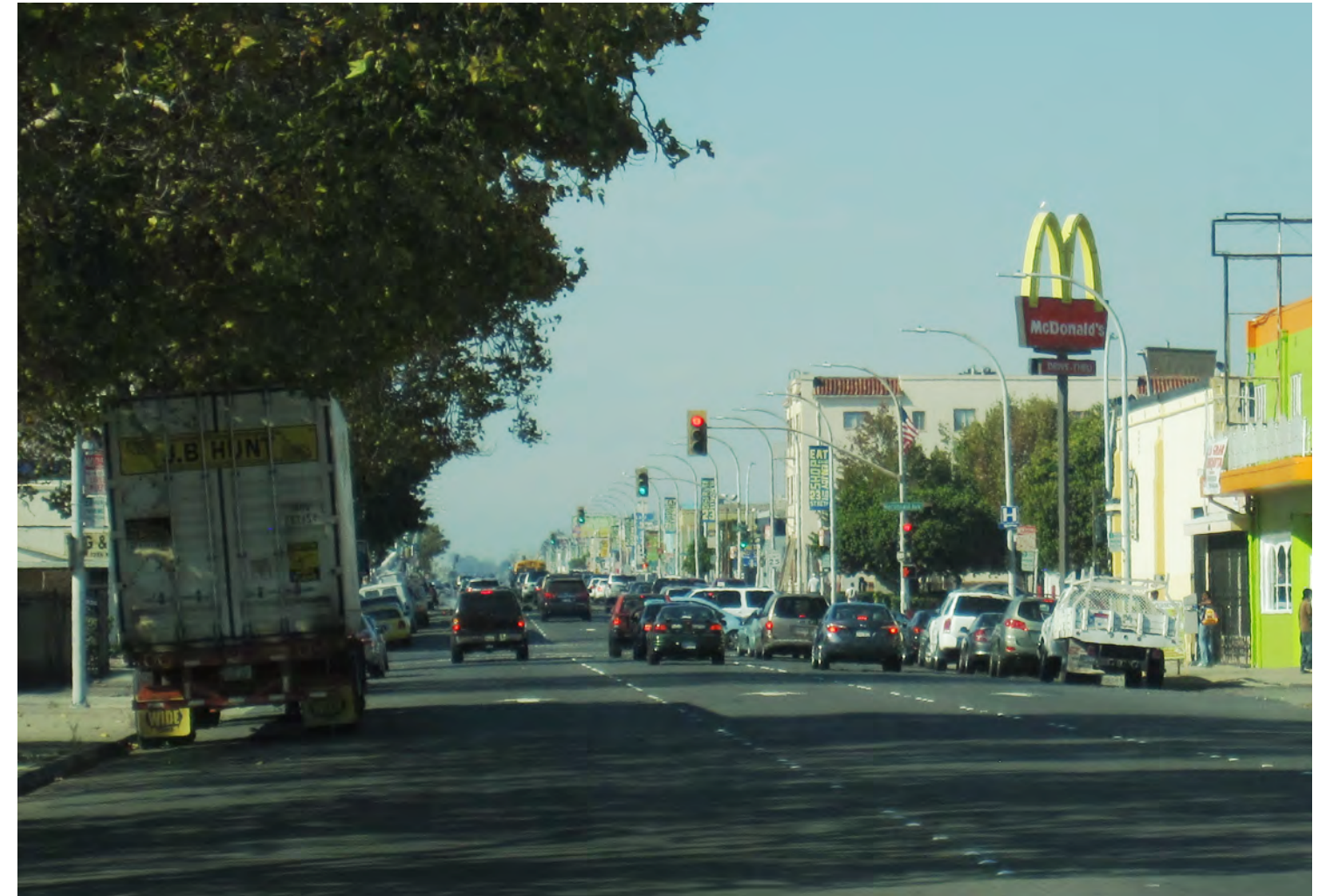
Traffic signals on 23rd Street in Richmond
