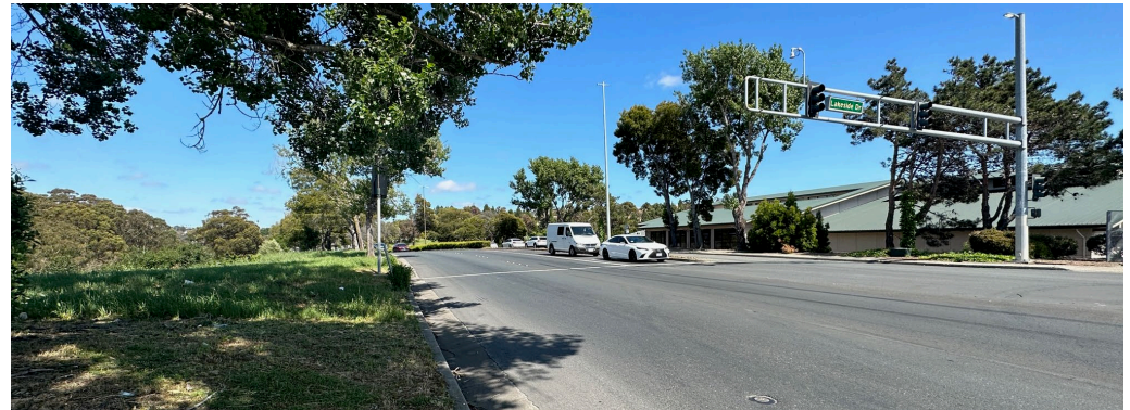
Missing sidewalks near more active land uses
