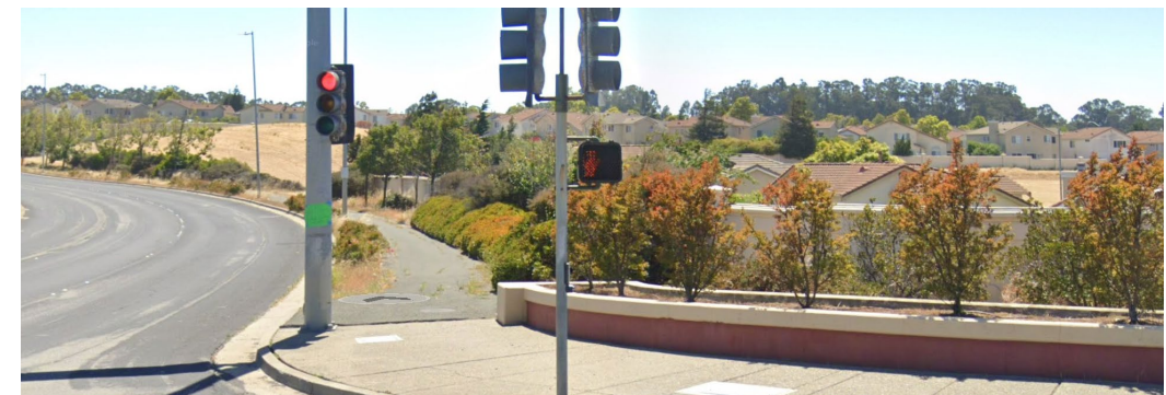
Limited signage indicating shared-use path
