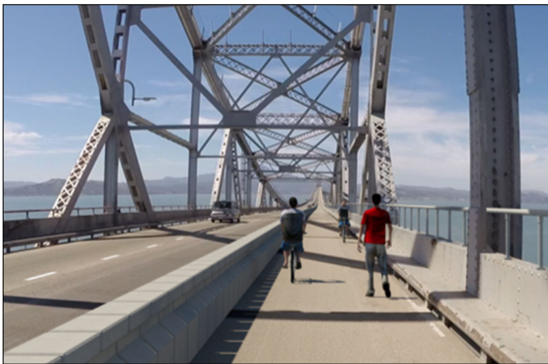
Above: A rendering shows the proposed 10-foot bi-directional bicycle-pedestrian path on the upper deck of the Richmond San Rafael Bridge. Path users will be separated from traffic by a movable concrete barrier system similar to the one installed on the Golden Gate Bridge in January 2015.
