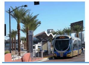
High-amenity BRT stations can include the following elements, as shown in this photo of Las Vegas' Max BRT system: landscaping, level boarding, ticket vending machines, distinctive station, maps and other wayfinding tools, trash can, and others
