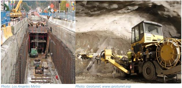
Excavated trench for cut and cover tunneling (left photo) and drilling machine (right photo)
