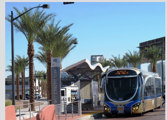
High-amenity BRT stations can include the following elements, as shown in this photo of Las Vegas' Max BRT system: landscaping, level boarding, ticket vending machines, distinctive station, maps and other wayfinding tools, trash can, and others.
