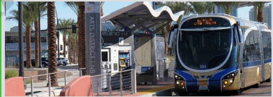
High-amenity BRT stations can include the following elements, as shown in this photo of Las Vegas' Max BRT system: landscaping, level boarding, ticket vending machines, distinctive station, maps and other wayfinding tools, trash can, and others.
