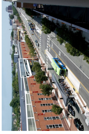
Directional center platform with right-hand boarding
