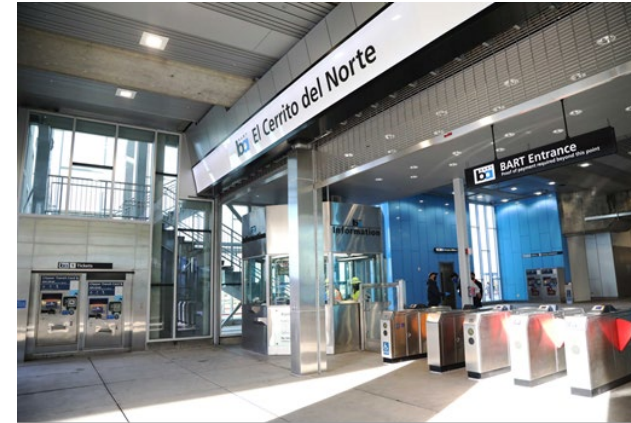
External view of fare gates
