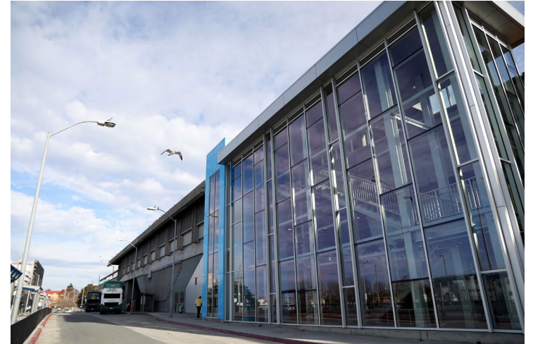
External station view
